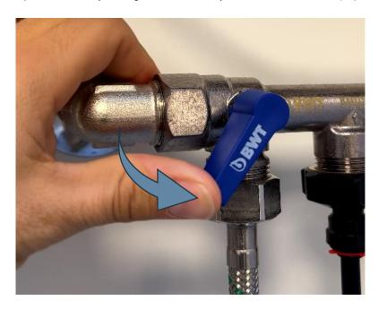
Check the installation for leaks before tuning the unit on.
