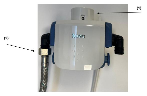
Mount a hose from the filter head outlet to the autoclaves.
