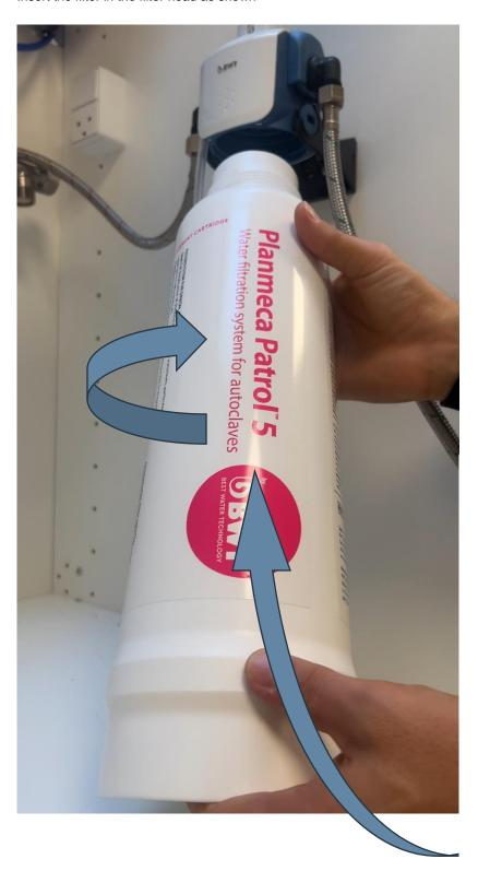
When the filter has been mounted in the filter head it needs to be flushed. Turn the little flush knob next to the bypass selector.
