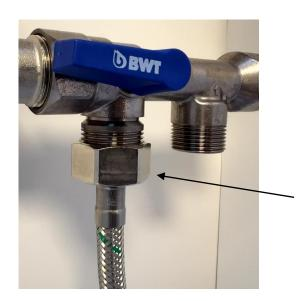
Mount the other end of the inlet water hose (15) on the Water Inlet (C).
